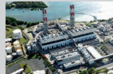
An aerial view of the WAPA power plants in the U.S. Virgin Islands
